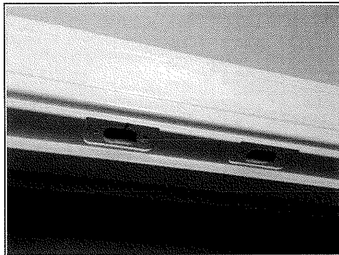
Ball catch strike plates for linen closet doors missing.
